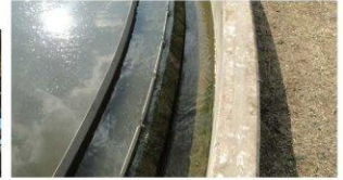
Chlorinator after 6 days.
