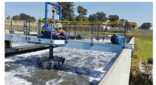
Aeration Basin before cleaning
