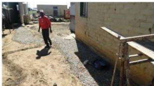
Yard drained and crusher stone laid to provide dry access to house
