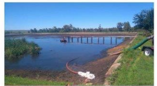
Inlet pond being cleaning
