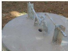
New lockable manholes installed
