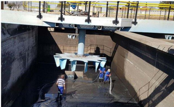
Cleaning the Aeration Basin
