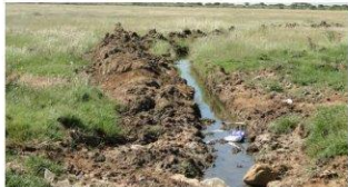
Existing trenches opened to divert sewage water
