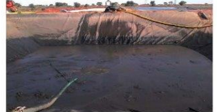
Inlet pond being cleaning
