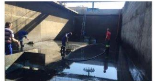
Cleaning the Aeration Basin
