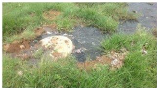
Sewer overflowing from manholes and running into fields next to the township.
