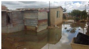
Flooded house before temporary intervention
